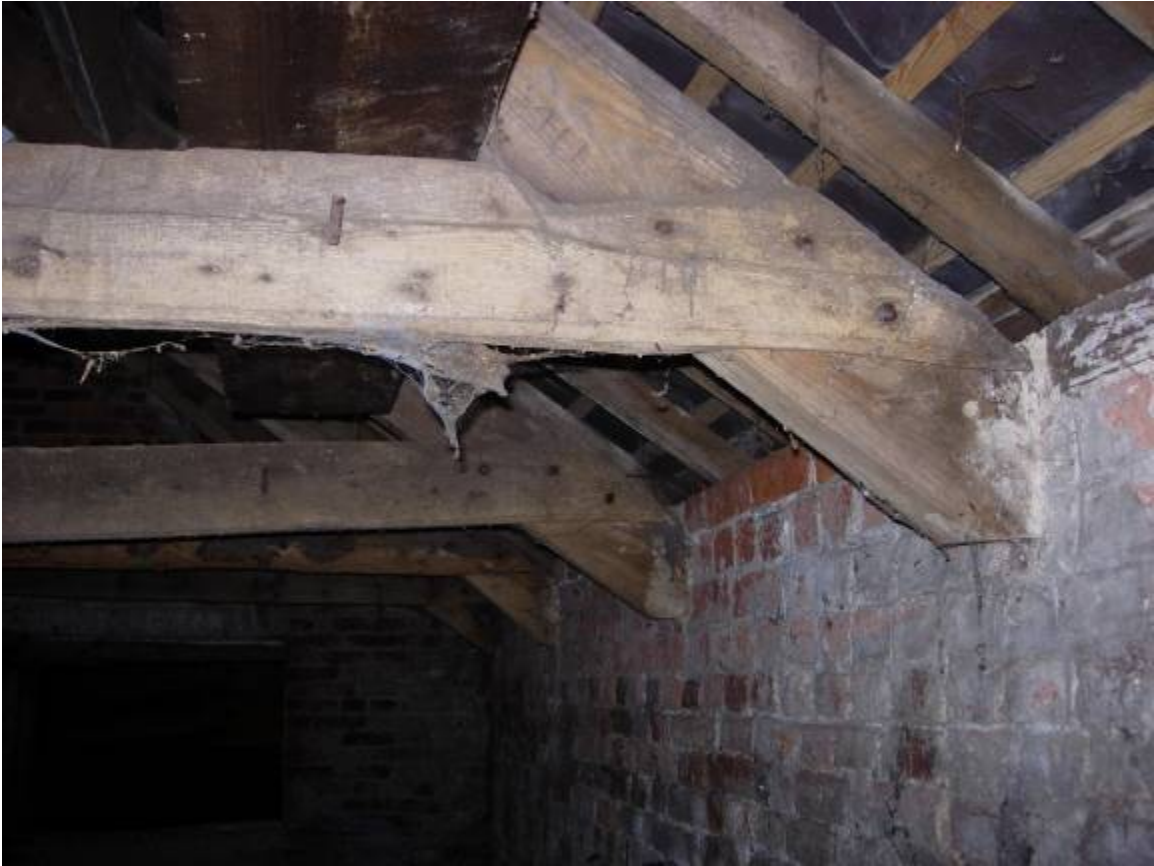
Earlier truss form showing assembly numbering in eastern part of potting shed range. 2013
