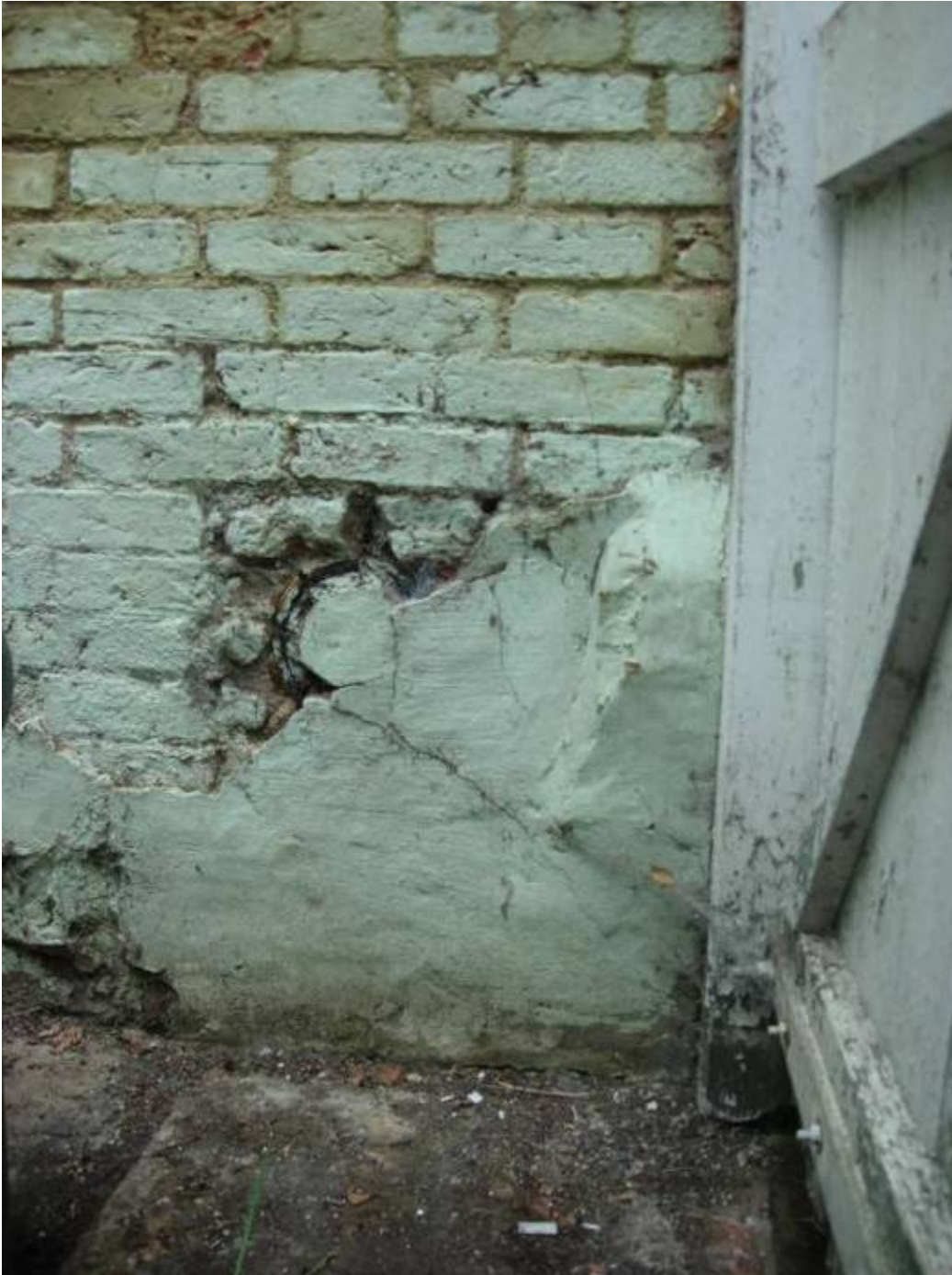
Stub of cast iron heating pipe at the east end of the range. Removal of render here would perhaps reveal another pipe below (providing flow and return) both perhaps set into an earlier flue opening (c.f. above photo of west end)
