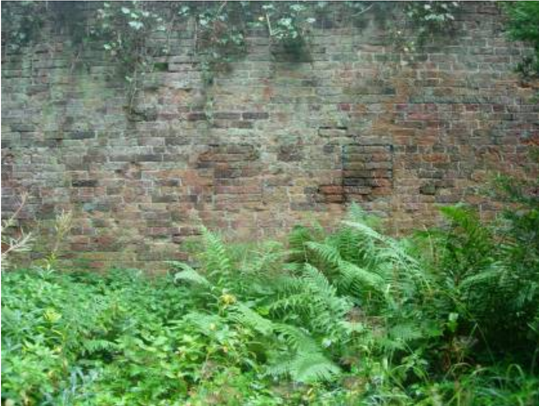
A number of paired openings can be seen on the north side of the garden wall, indicating removable brickwork to allow access for cleaning the flues of the hot wall
