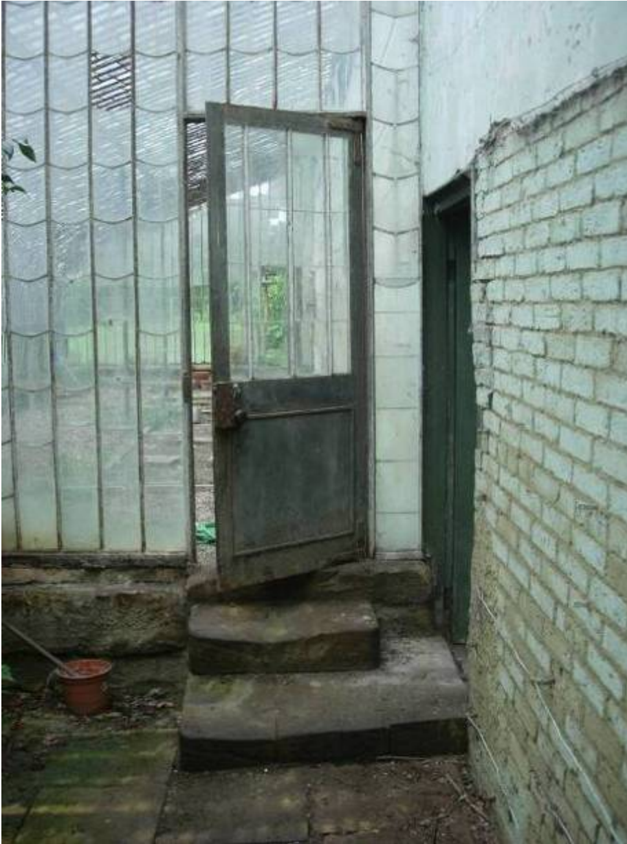
The well worn steps at the central partition suggest a long period of use. The heavy iron partition door is harr-hung, turning on pintles top and bottom. 2013
