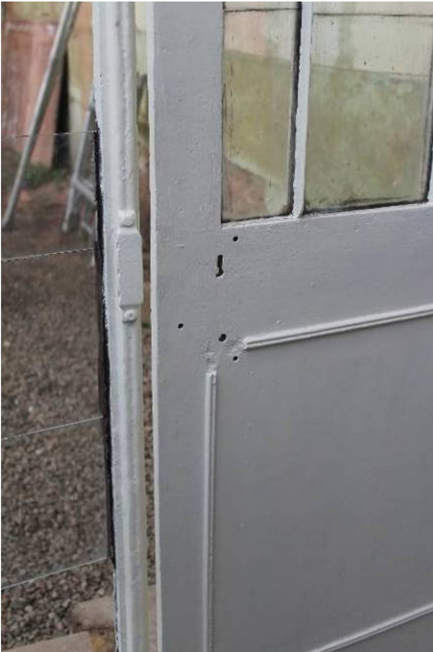
Partition lock box removed during repairs 2015. N.B. the moulding on the cast iron door plate was cut away to accommodate the lock, indicating that the lock was not part of the original design
