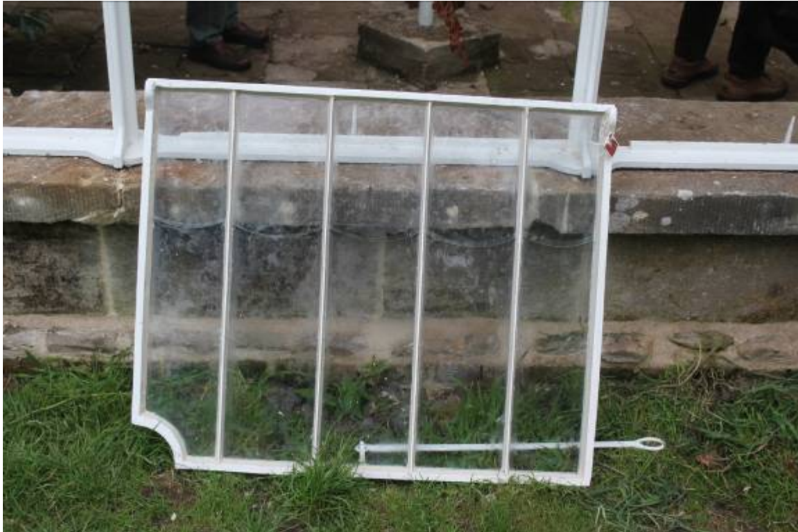
Restored casement from eastern division showing stay to control degree of opening (locating pin on sill behind) and rebate for vine stem to pass into the house from an external vine border
