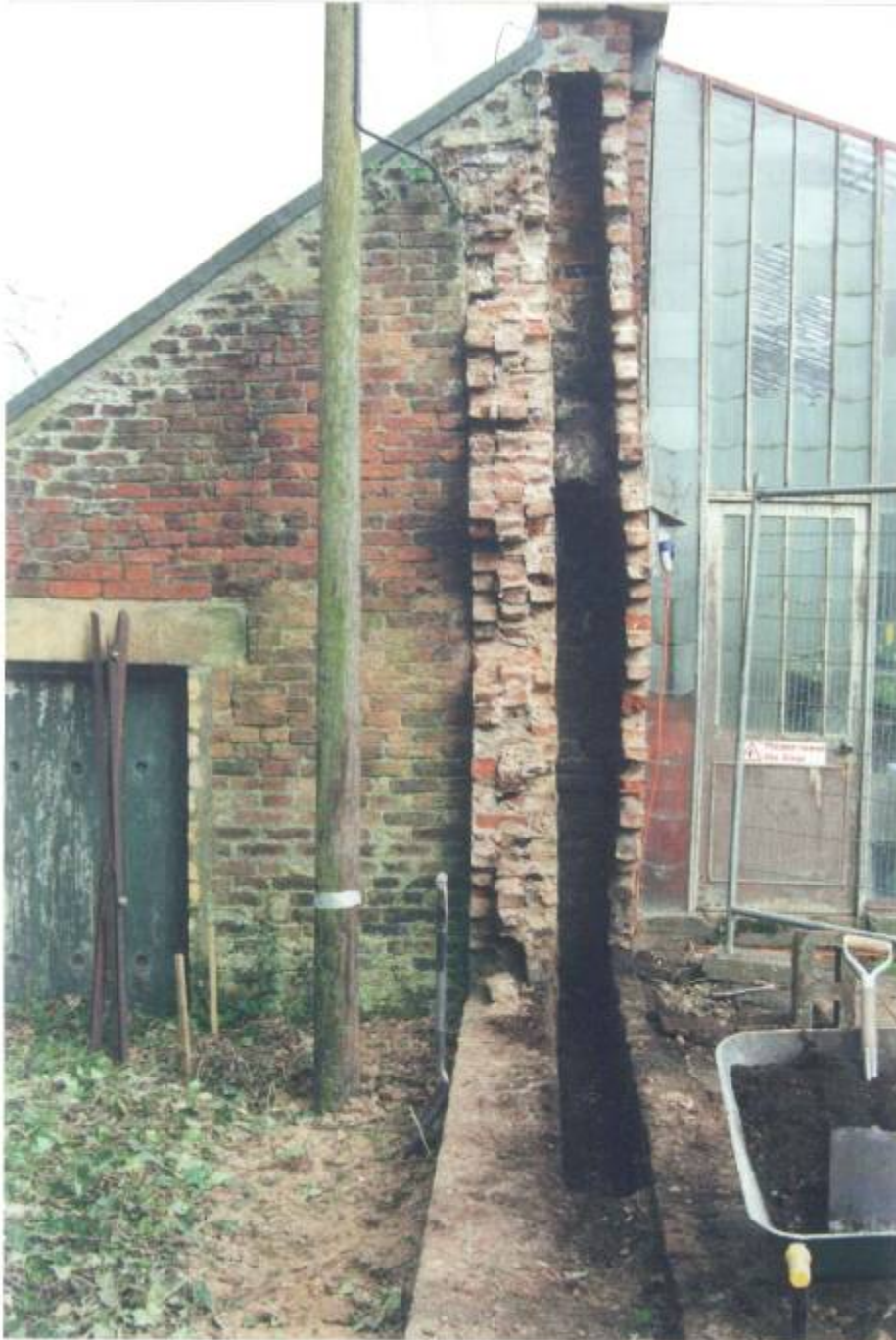
The garden wall to the west of the glasshouse was heated by internal flues, seen in section when the wall was dismantled for repair in 2002. The offset to accommodate the glasshouse can be seen at the wall head. [Photo. Robin Dower]
