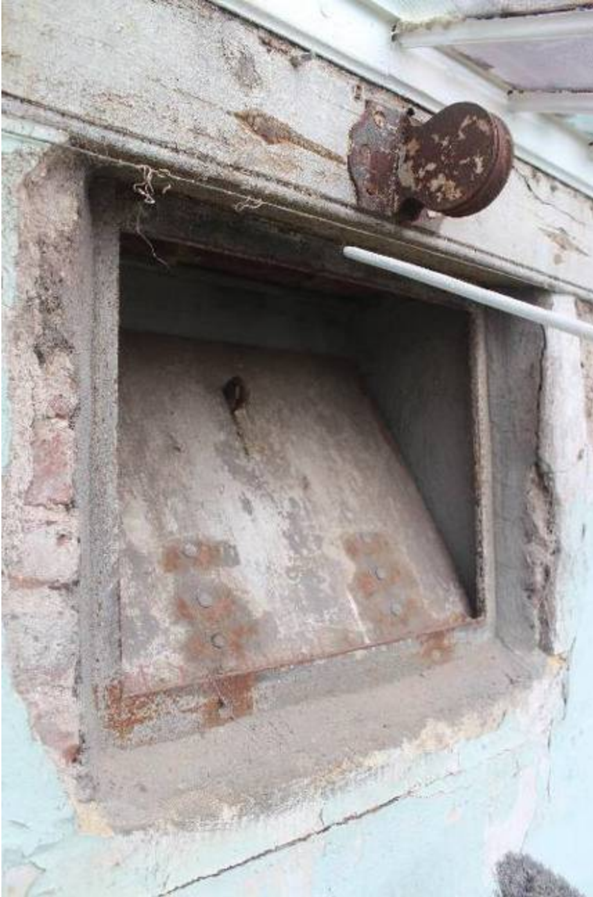
Ventilation opening at the top of the back wall. The arrangement for notching the top of the glazing bars over the top rail can be see top right
