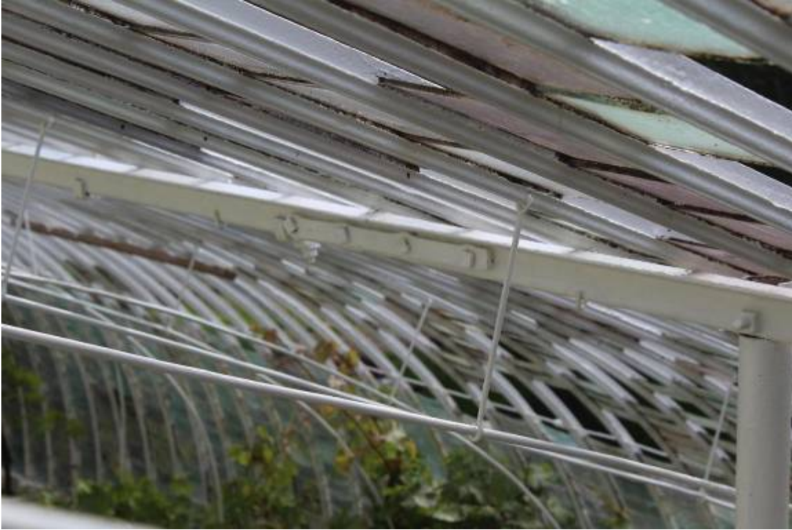
Fish plate joining sections of the purlin in the eastern part of the range. Note clips securing glazing bars to the purlin and arrangement for hanging the vine training wires from the glazing bars
