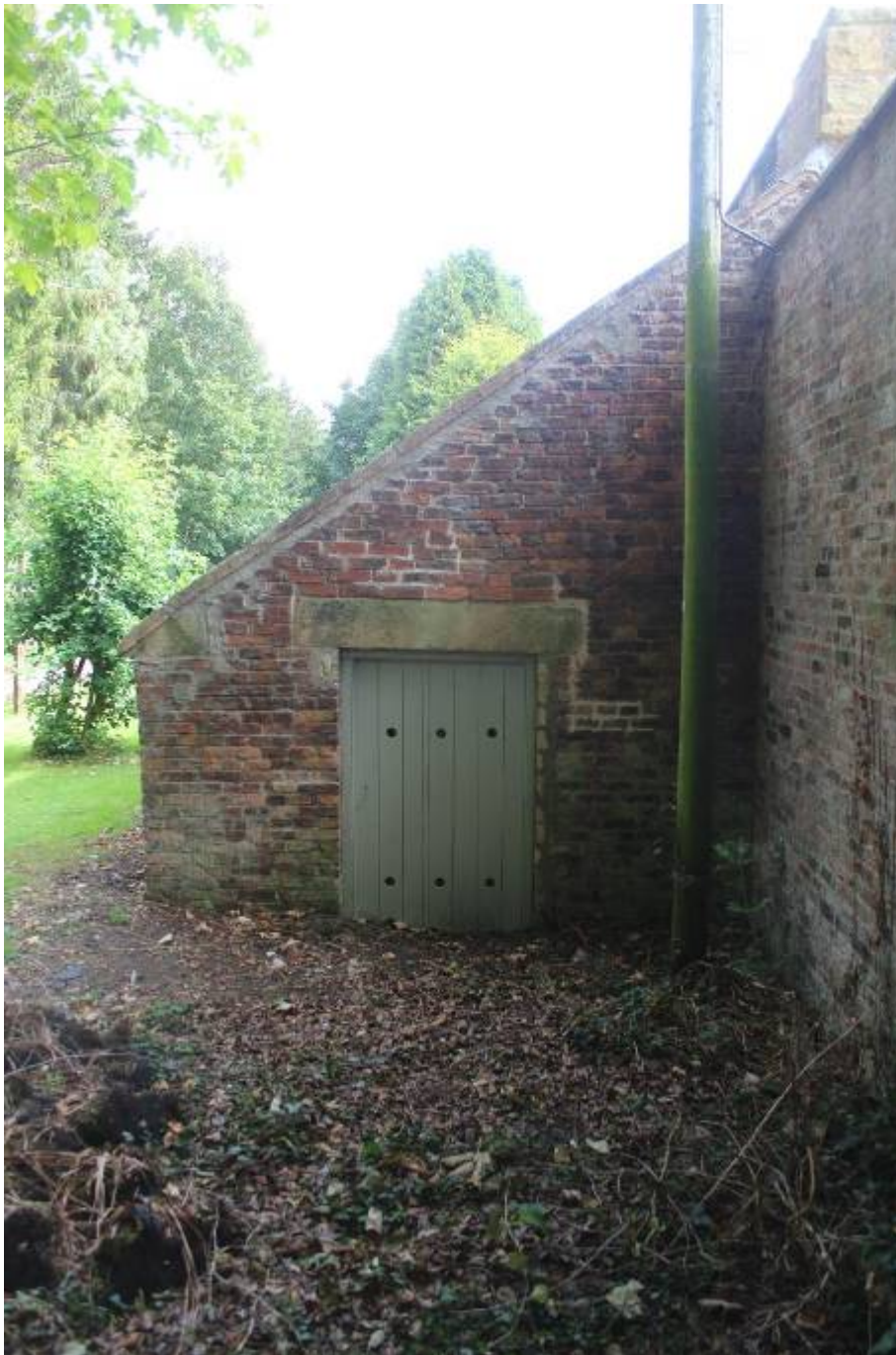
The west end gable brickwork suggests a rebuild of the upper courses, perhaps to accommodate the lifted roof of the potting shed
