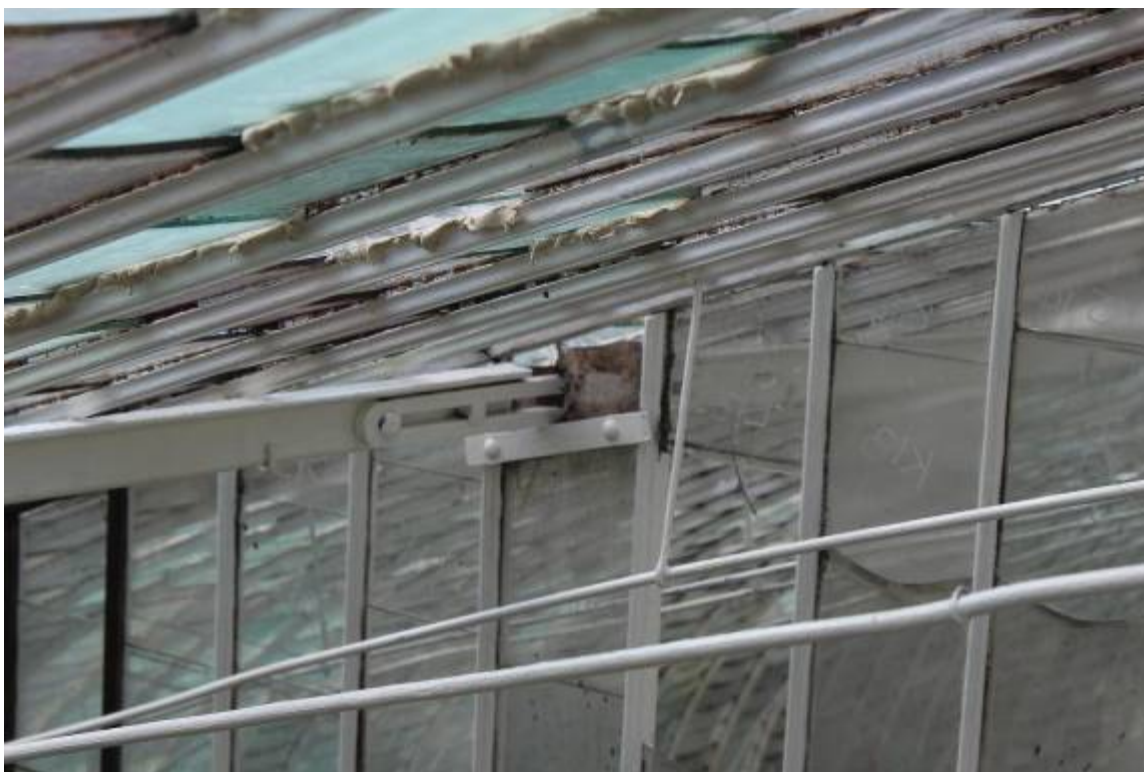
The support purlin passing through the internal partition. The join here may have been designed to accommodate thermal movement of the purlin. Sept 2015
